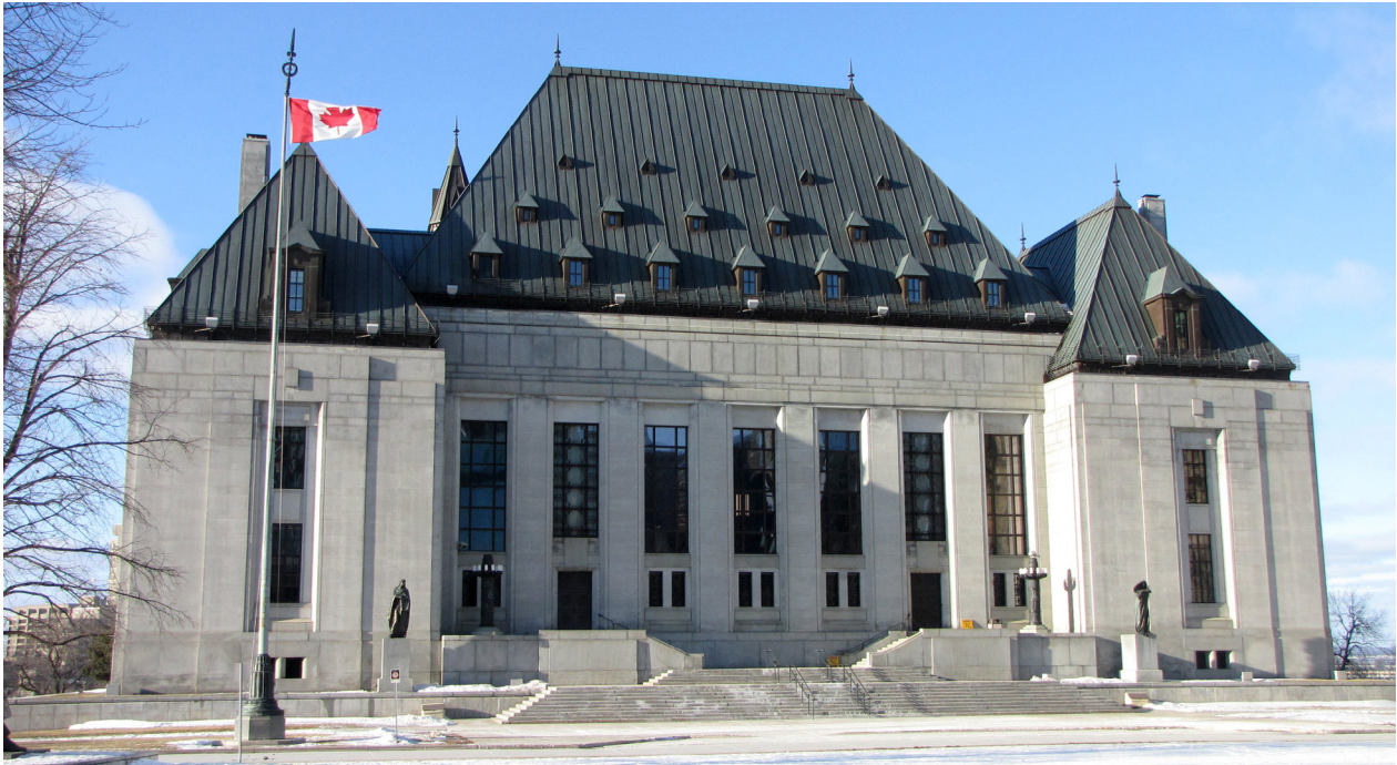
Supreme Court of Canada Building Ottawa, Ontario, Canada
